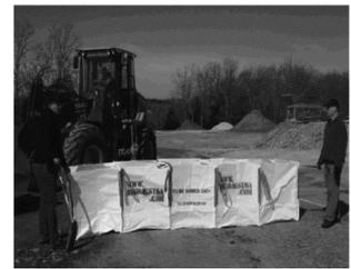
Try this: Using one ground crew to attach systems while two other ground crews expand Big Bags USA systems will enable continual deployment for a fast response time.
